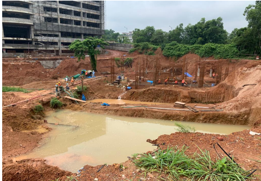
Building 2 under construction
