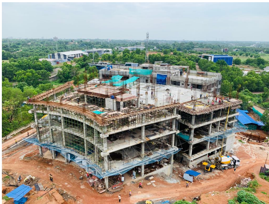
Building 1 under construction
