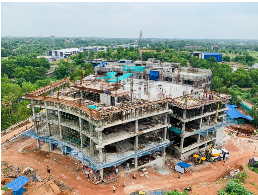
Building 1 under construction
