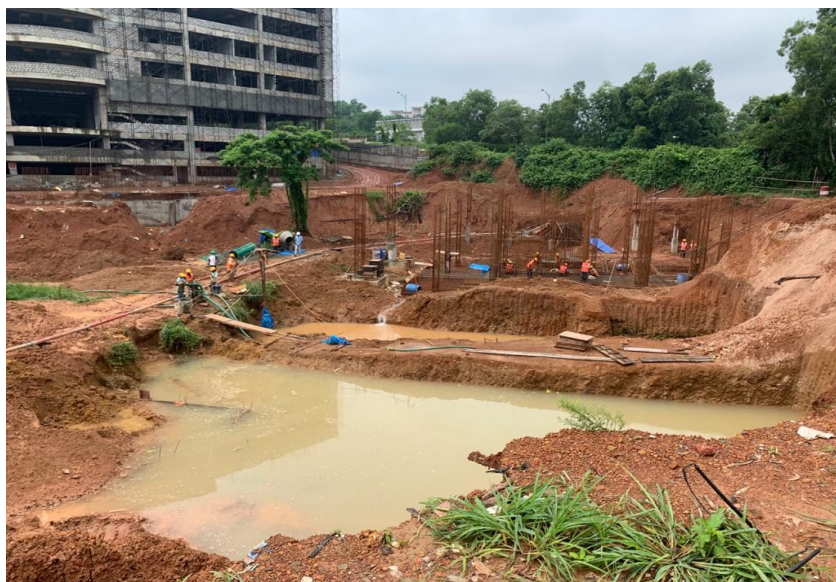
Building 2 under construction
