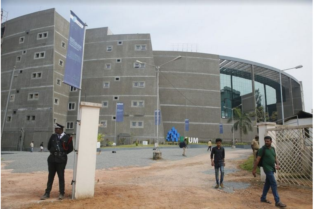
Integrated Start-up Complex
